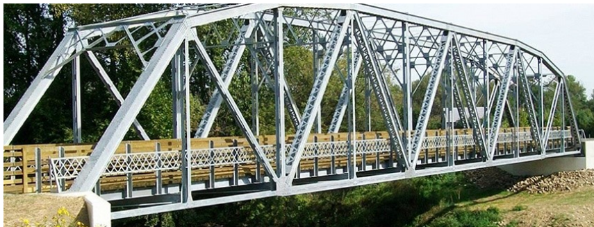
A Truss Bridge
